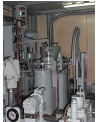
Before Retrofit - Hitachi Mechanical Cabinet Actuator
