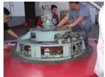
Mechanical Over-speed Device on top of PMG, to be replaced by L&S SSG
