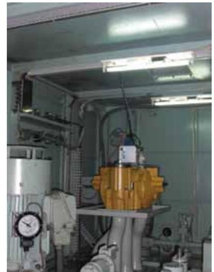
After retrofit - L&S Manifold & Distributing Valve mounted in the existing governor cabinet
