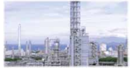
Chandra Asri Petrochemical Plant
