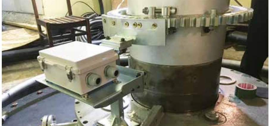
PMCS Designed Speed Gear and MPU Mounting
